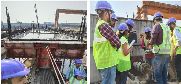
Precast Girder Workshop
